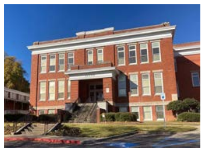
Adaptive Reuse of Existing Historic Building
